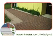
Porous Pavers: Specially designed paving stones, bricks, or pavers allow water to soak into the ground below.
